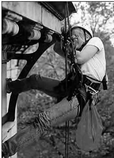
Susan Knack, a civil engineer for Simpson Gumpertz & Heger, rappels down buildings to examine its construction for various problems or conditions.
